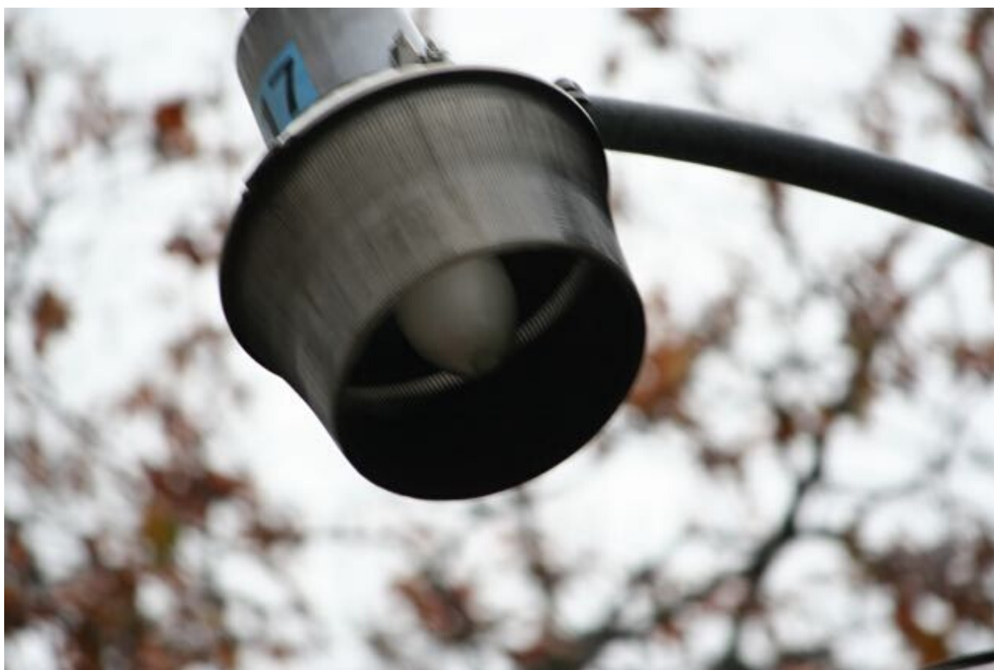
BARNYARD LIGHTS SUCH AS THIS ARE LESS THAN 30 PERCENT EFFICIENT, SENDING MOST OF THEIR LIGHT OUT IN THE GLARE ZONE OR UP INTO THE SKY. MANY, IN CONSEQUENCE, ARE PAINTED BLACK TO AVOID THROWING MISDIRECTED LIGHT INTO NEARBY HOMES.
